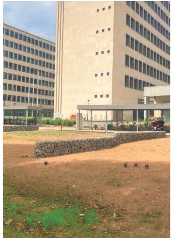
Figure 40 - Murets en gabion
